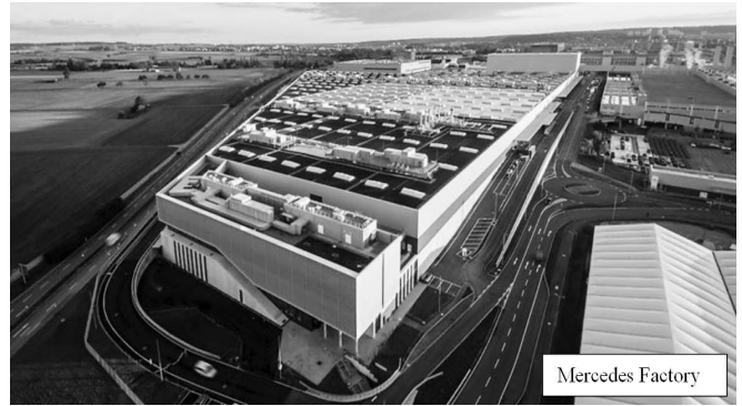
Figure 2. World’s first captive 5G mobile network has been installed for automobile production over an area of more than 2 million square feet.
