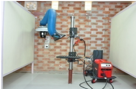
Trans Steel Welding Station
